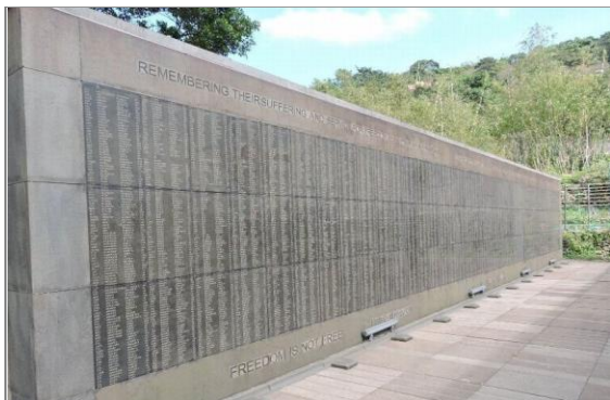
The restoration of the POW Memorial Wall.
